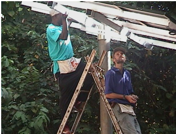
Figure 23. Installation of the new solar panels (left) and satellite dish (right) (25 May 05 and 08 Dec 05; MLW)
