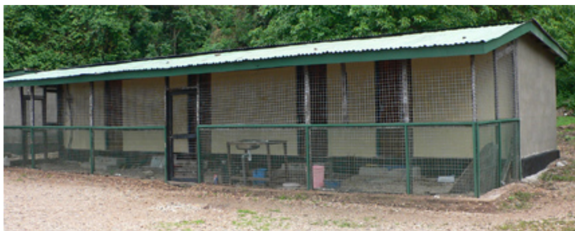
Figure 22. Staff quarters in Kasekela: new paint, doors, sinks, and roofing. (23 Nov 05; MLW)
